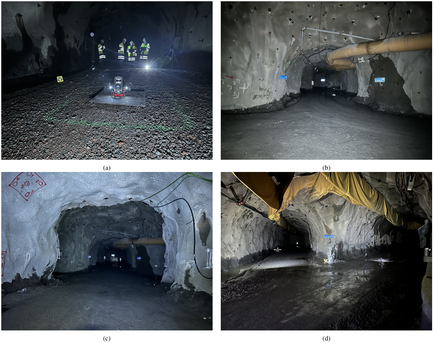
Fig. 14: Pictures showing the mining environment where the system was deployed and evaluated. (a) shows one of the aerial agents used to perform the inspection tasks prior to takeoff, (b) – (d) shows three snapshots of the tunnels in the underground mine where the evaluation mission was performed.
