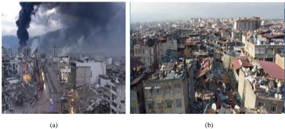
Figure 22. Drone Captured Images (a) Collapses in Iskenderun on both sides of the road; the amount of obstruction is much larger than a 45° angle may suggest. (b) Partial building dismantled in Hatay, requiring total demolition (with copyright permission from PEMA [226][227])
