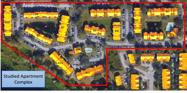
Fig. 1. Potential useful solar panel installation areas for studied apartment complex (Google Sunroof).
