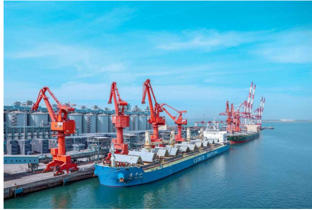
Figure 19: A number of cranes working simultaneously at Qingdao Seaport.
