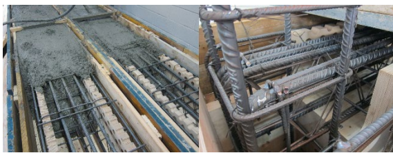
Fig. 4 Concrete pouring in simply supported and frame-connected beams.
