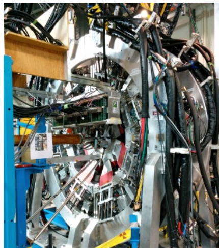
FIGURE 2.8: Installation of TIGRESS in Experimental Setup
