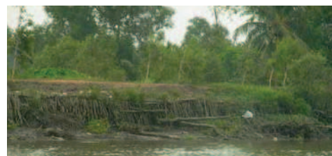
Figure 2 Countermeasure by wood piles
